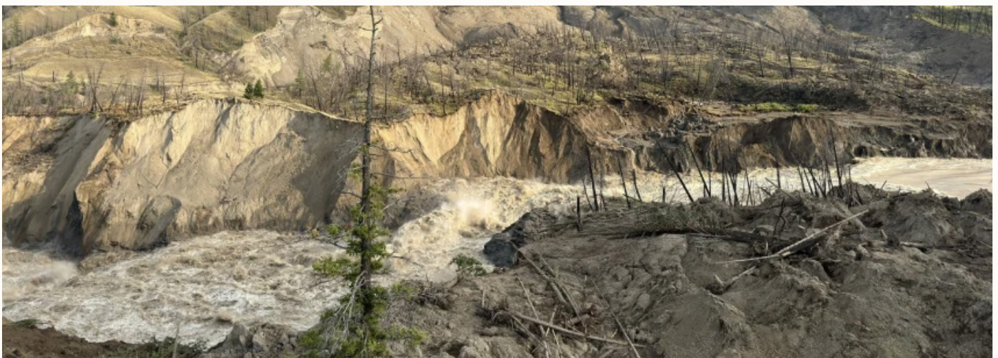
Roughly six hours after the dam breached, the Chilcotin River had cut a deep channel through the landslide debris. In the background, the landslide scar is visible on the slope as a lighter, sandy area surrounded by greener foliage and blackened tree trunks. Photo by Brian Menounos
